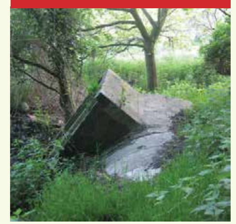
Remains of one of the air raid shelters.
