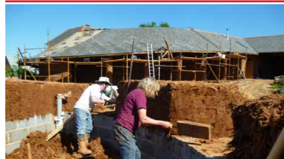
Playing in the mud: a new cob building is created.
