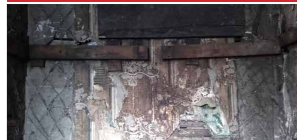
One of the most exciting surviving elements is the presence of a 18th and 19th centuries wallpaper laminate found in a cupboard of a principal room of the building fronting onto the street.
